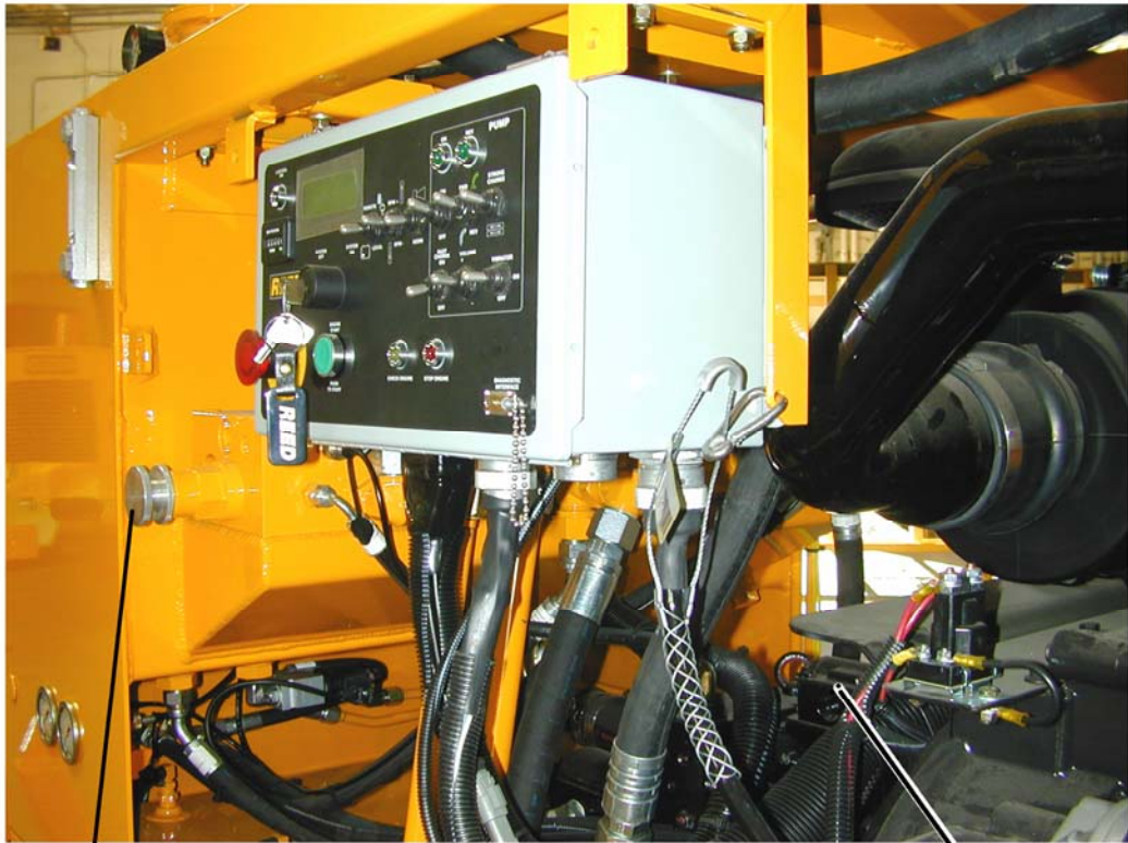
CONTROL BOX WITH COVER REMOVED
