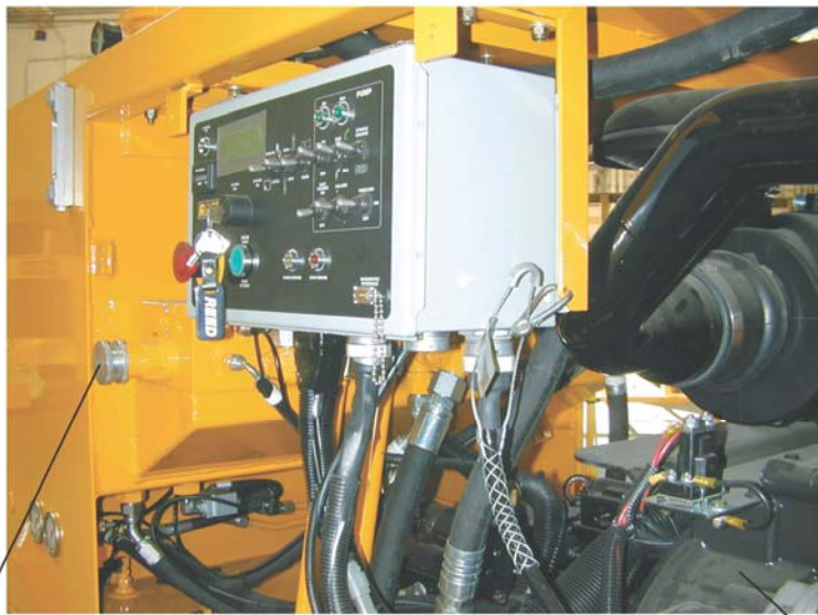
CONTROL BOX WITH COVER REMOVED
