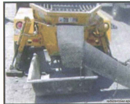
Figure 25 Cover reducers and use containment boxes for cleanout
