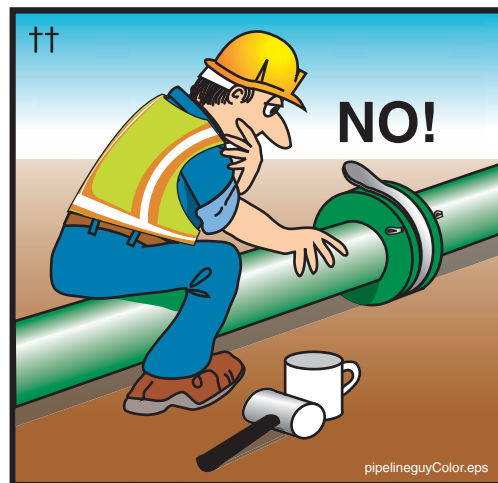
Figure 50 Never straddle or sit on a pressurized pipeline
