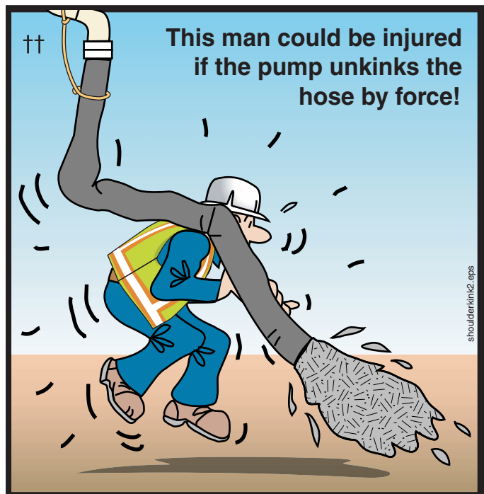
Figure 86 Never kink the hose; Never hold the hose with your shoulder
